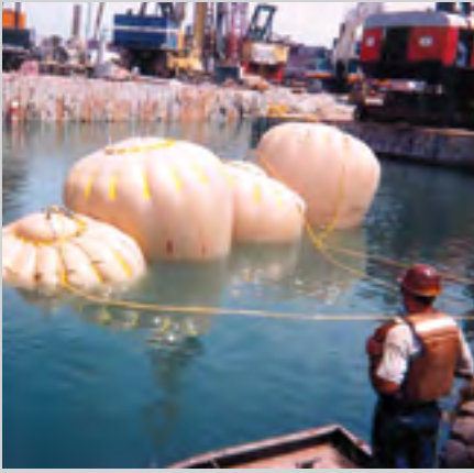
Professional lift bags used to lift a 100 ton concrete abutment during the Big Dig tunnel construction in Boston.
