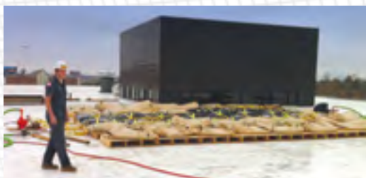
Roof load testing using Enclosed Water Weight Test Bags.
